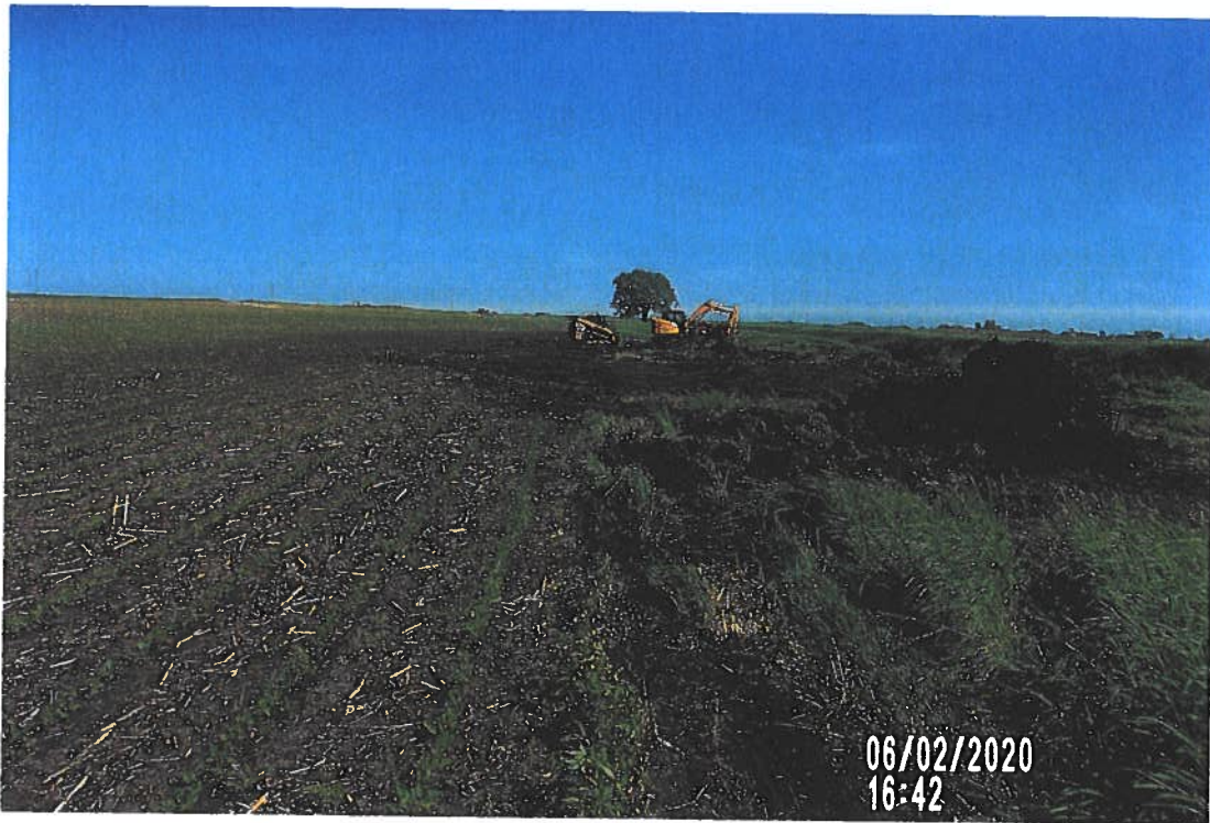
PICTURE #3641 IS LOOKING SE AT 0.14' AC OF BEAN DAMAGE DURING REPAIR
