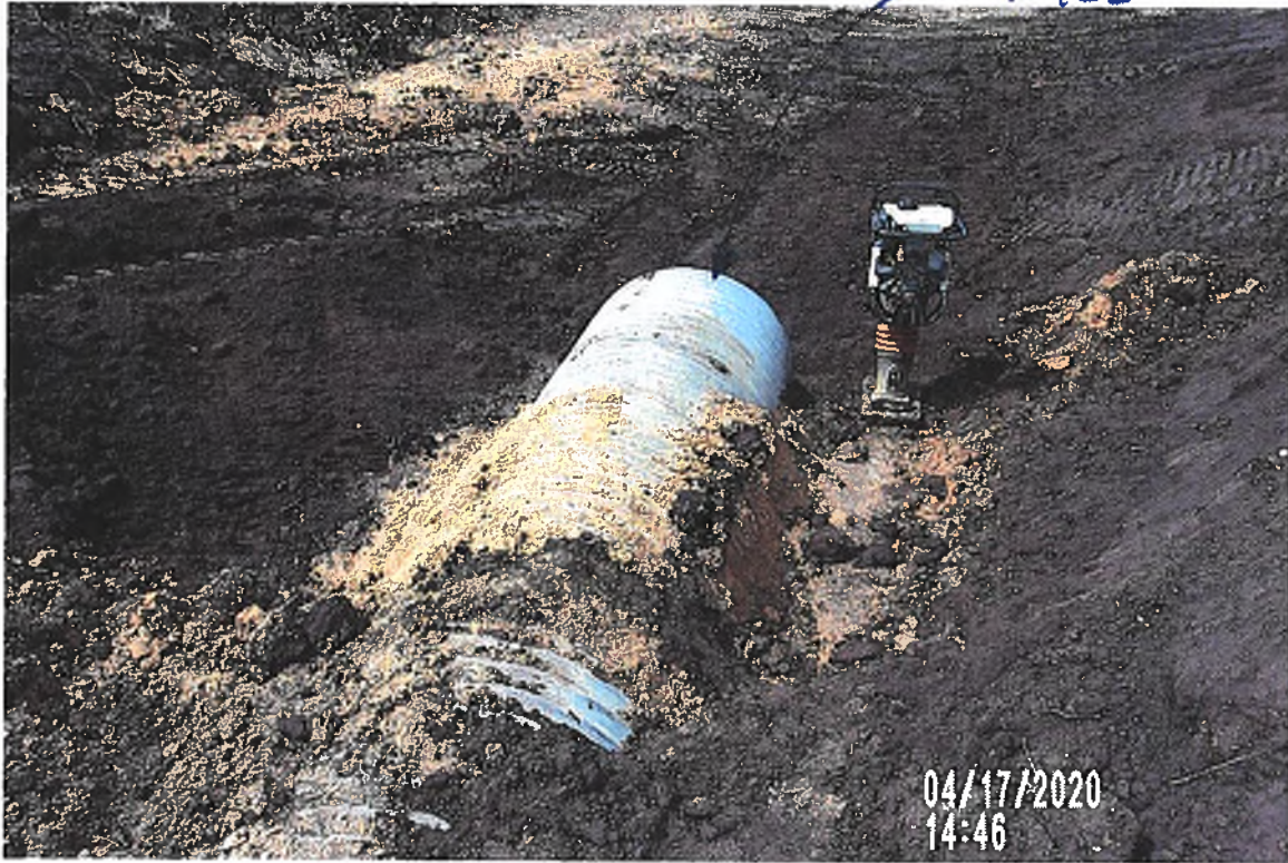
PICTURE# 3390 IS LOOKING NW SHOWING CREW STILL JUMPING JACK COMPACTING BACKFILL SOIL ON NORTH END OF 36" CMP SURFACE DRAIN. / GPS#428
