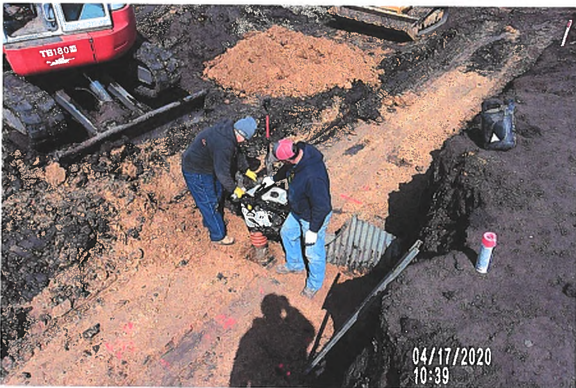
PICTURE # 3374 IS LOOKING NW SHOWING CREW VIBRATORY PLATE COMPACTING BACKFILL SOIL AROUND METAL ANTISEEP COLLAR BEFORE SURFACE DRAIN INSTALLED.
