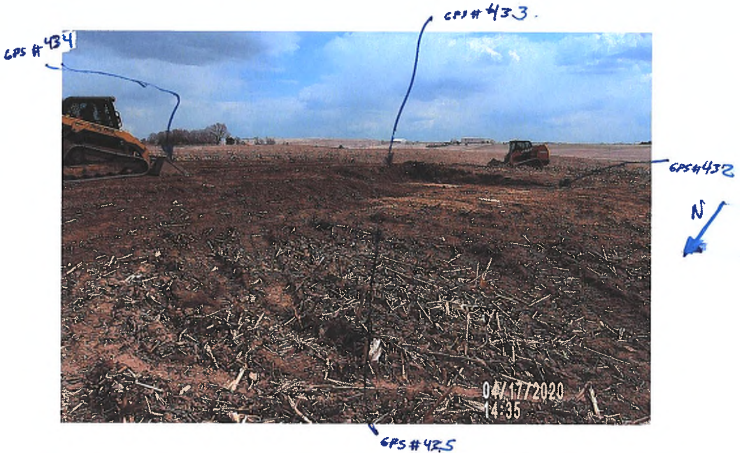
PICTURE # 3388 IS LOOKING SE SHOWING CREW DRESSING UP BORROW AREA.
