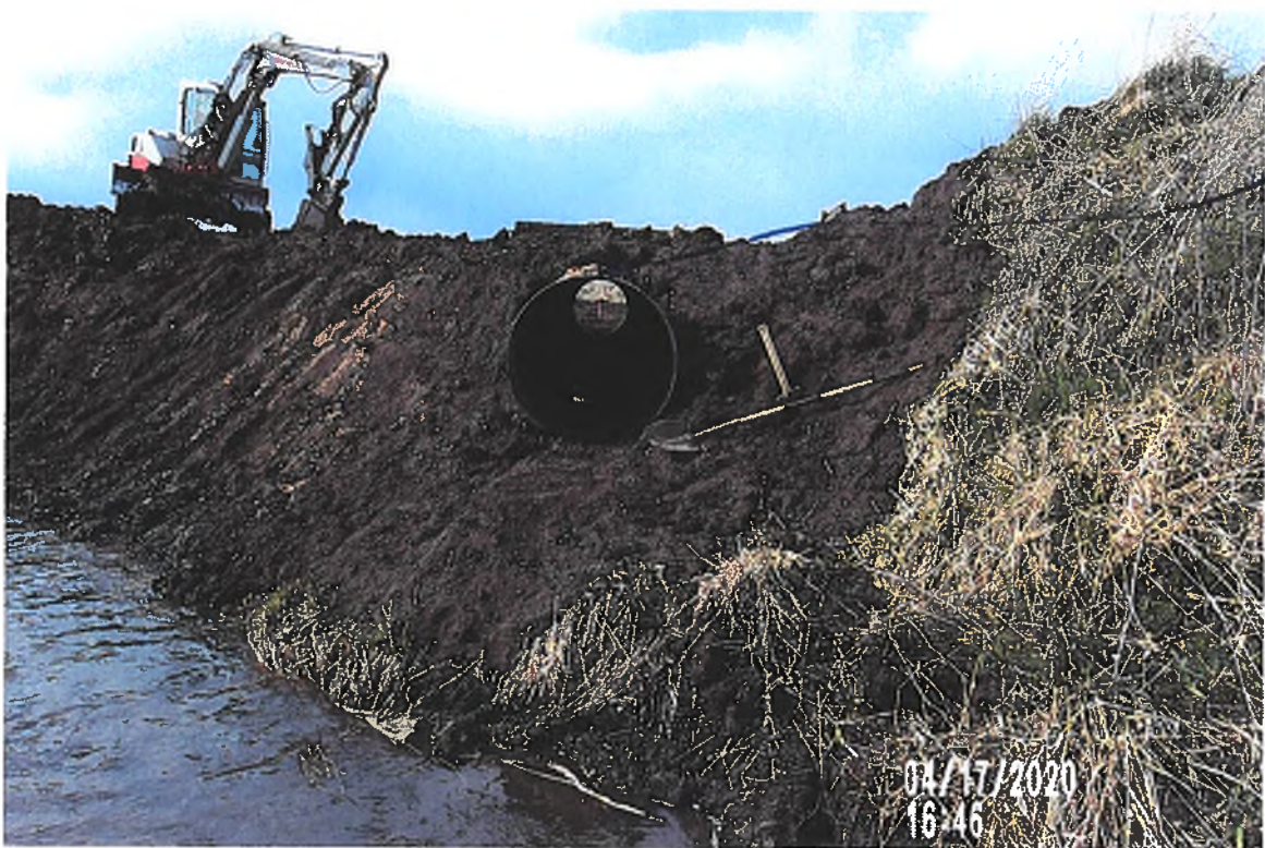
PICTURE# 3391 IS LOOKING NW AT DRAINAGE DITCH BANK GETTING BACK FILLED AROUND 36" CMP SURFACE DRAIN.
