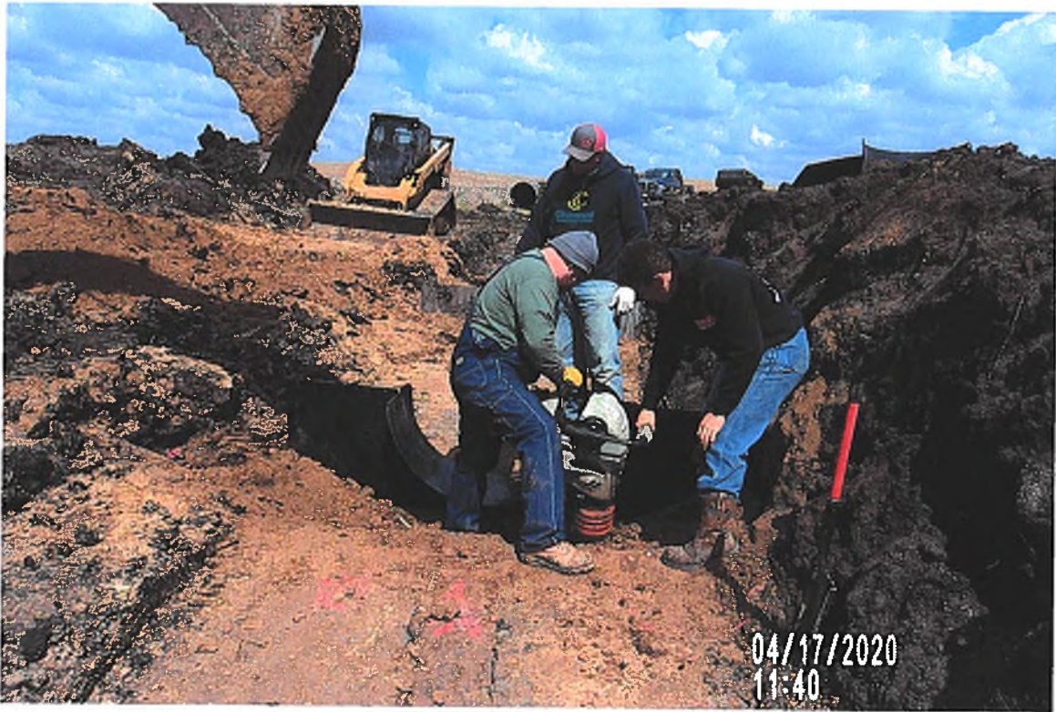
PICTURE # 3376 IS LOOKING NW SHOWING CREW VIBRATORY PLATE COMPACTING AROUND HDPE ANTISEEP COLLAR
