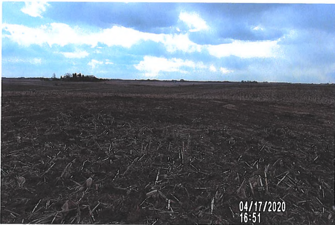
PICTURE # 3399 IS LOOKING SW AT BORROW AREA BACK FILLED AND DRESSED UP.
