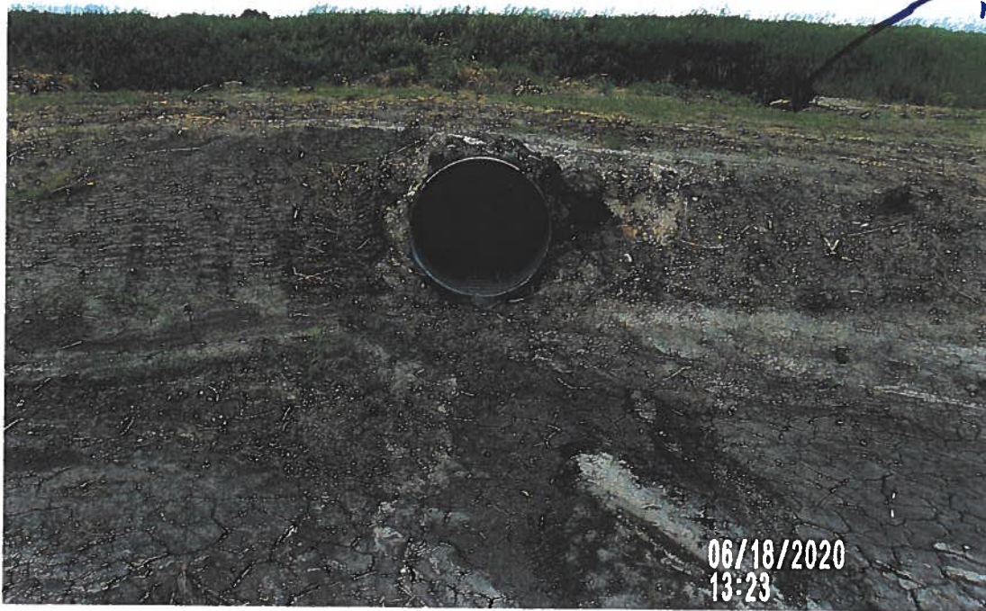
PICTURE # 3838 IS LOOKING SW SHOWING SOIL STARTING TO ERODE UNDER INLET OF NEW 24" CMP INLET. AND GRASS NOT GROWING.
