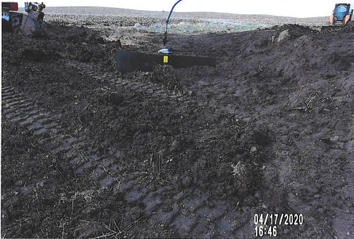
PICTURE#3393 IS LOOKING NW SHOWING CREW BACK FILLING DRAINAGE DITCH BANK AROUND CMP SURFACE DRAIN & AROUND HDPE ANTI SEEP COLLAR.
